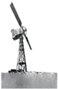
1941: Putnam's 1.25 megawatt turbine demonstrates the need for lighter materials
