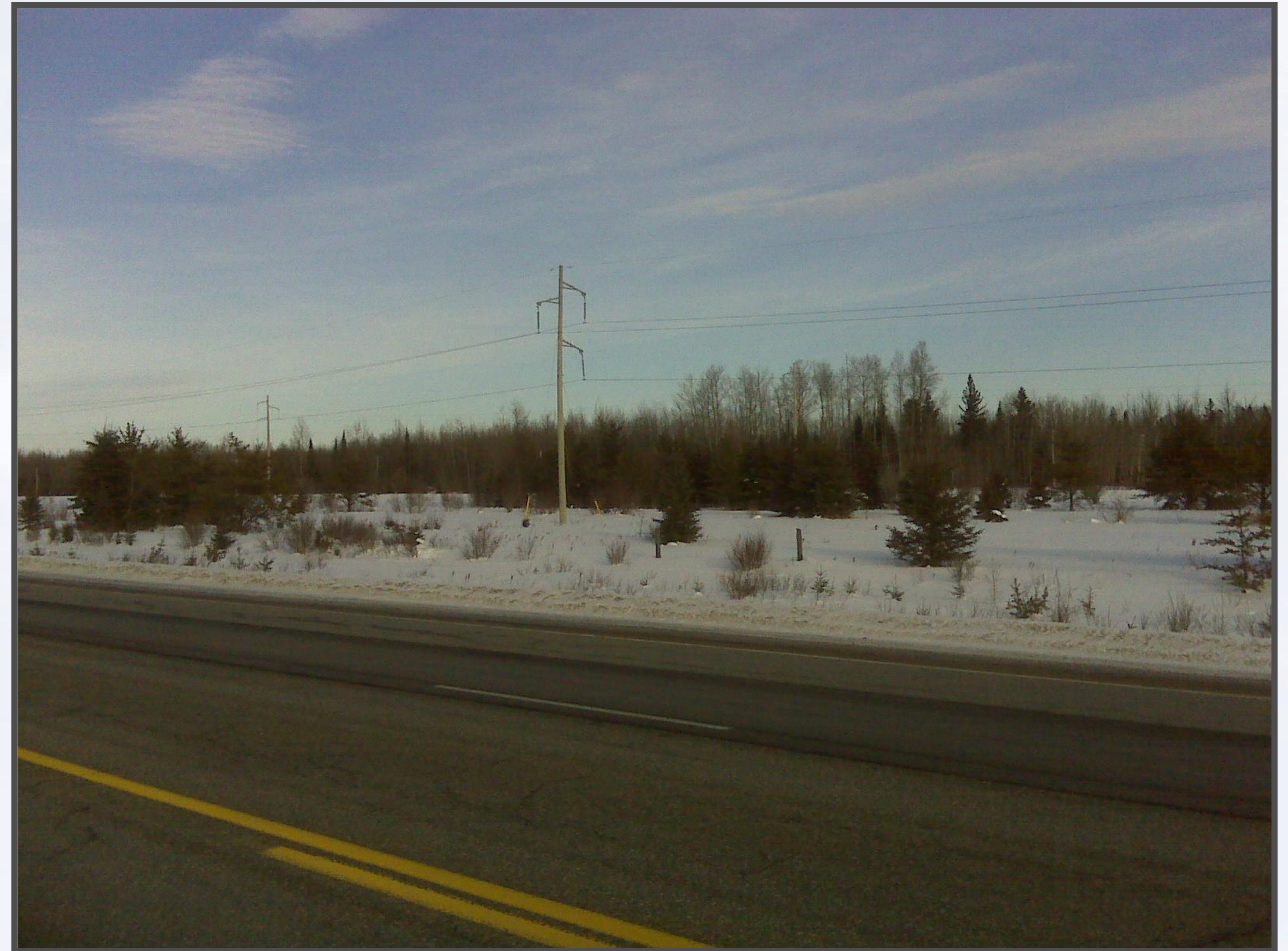
Typical single pole 115kV structure
