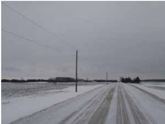
Both photos show existing infrastructure along the transmission route.
