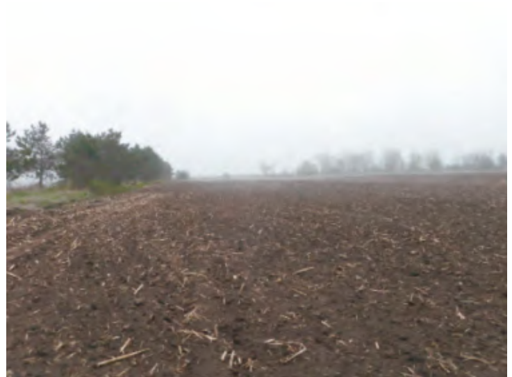
Plate 2 Turbine 1 Pad, View East (May 4 2012)
