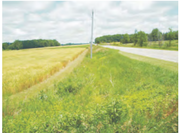
Plate 46 Proposed Transmission Line North Side of Road 183, View Northeast
