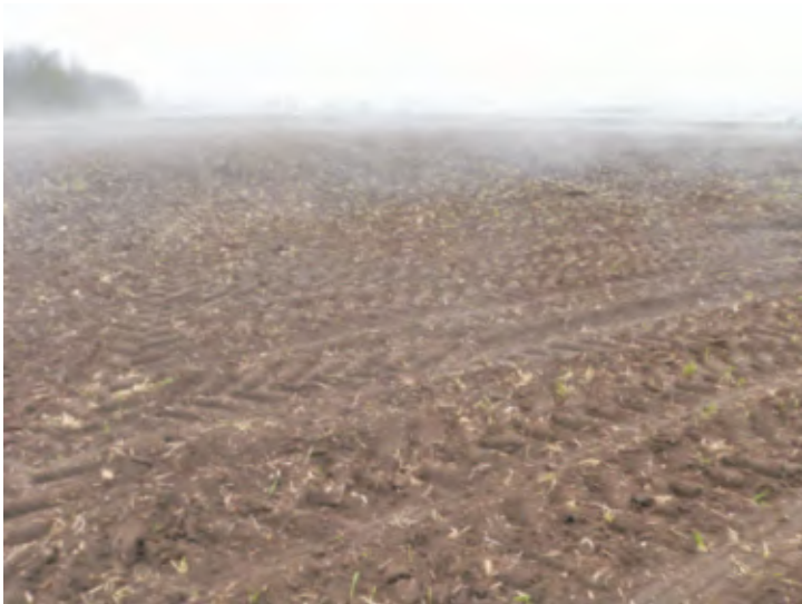
Plate 19 Turbines 29 Pad, View Southwest (May 4 2012)
