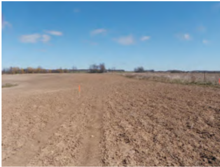
Plate 3 Turbine 3 Access Road, View East to Turbine Pad (April 5 2012)
