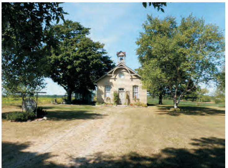
Plate 6 Former Schoolhouse on Blackbush Line, View West
