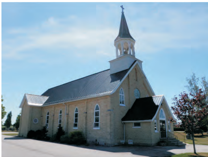
Plate 5 St. Peter's Catholic Church, View Southeast
