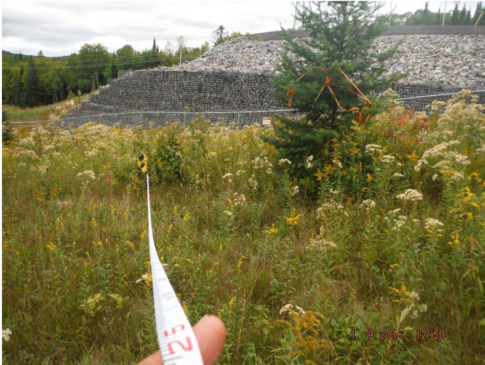
Figure 3 Looking Westward towards Substation along Transect C
