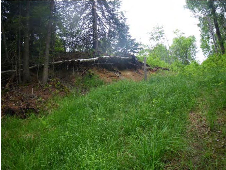
Figure 4.9 View of Groundwater Seepage Area on Slope Adjacent to Tributary A
