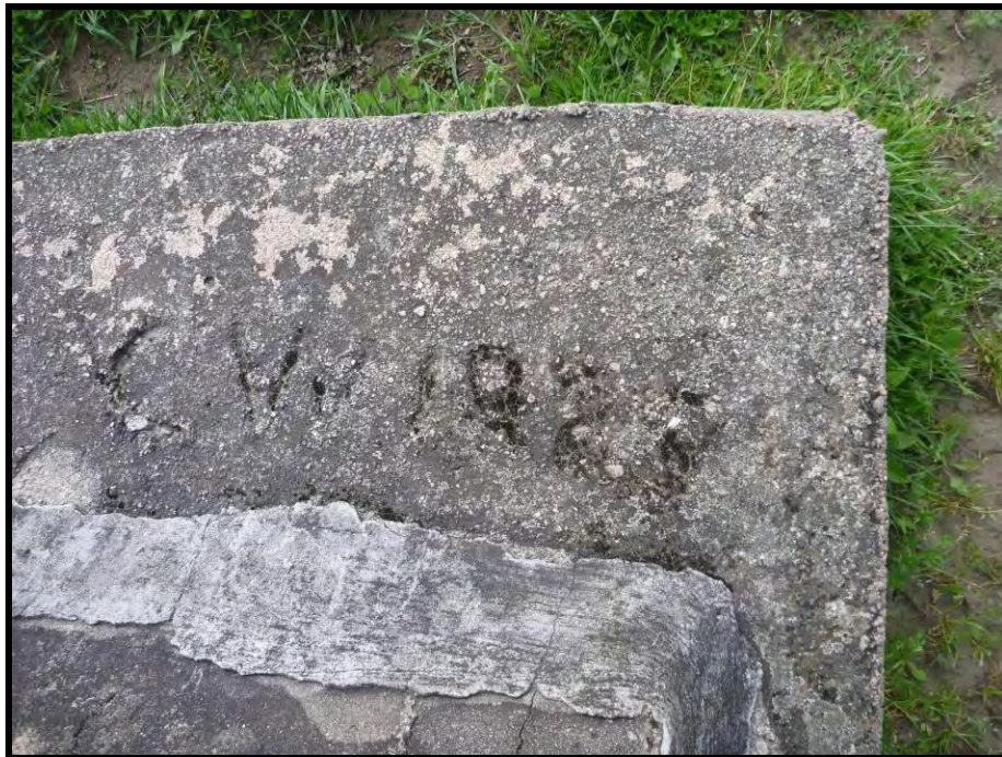
Plate 10: Detailed View of Cement Well Covering in Lot 13, Facing West
