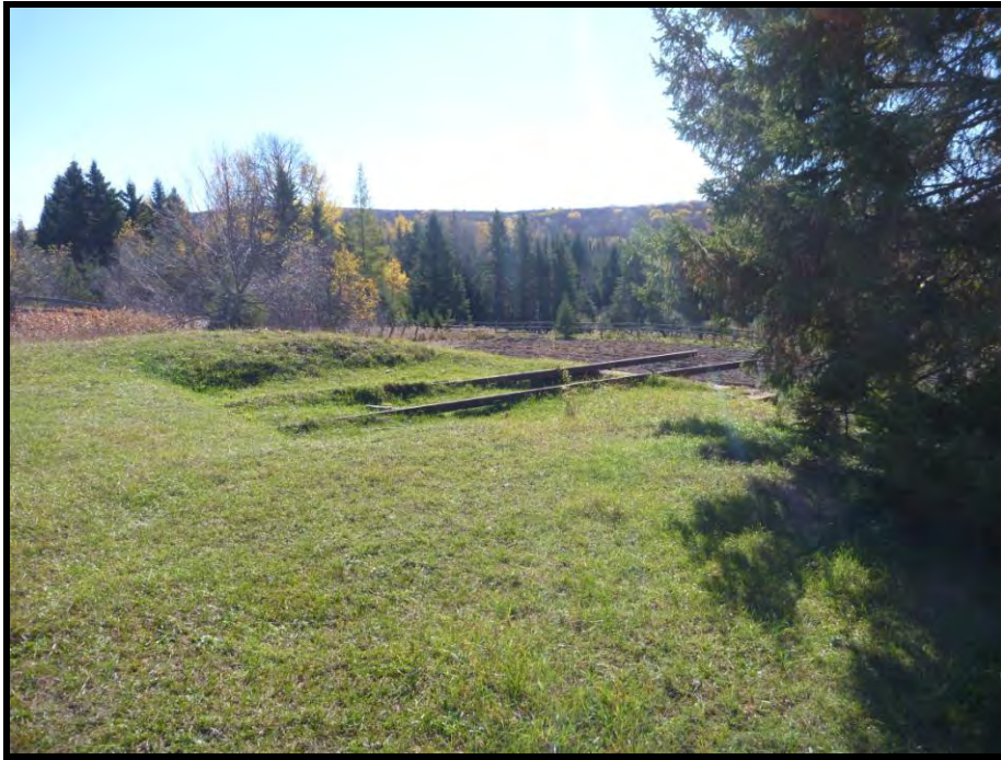
Plate 15: View of Concrete Foundation Outline, Facing Southeast
