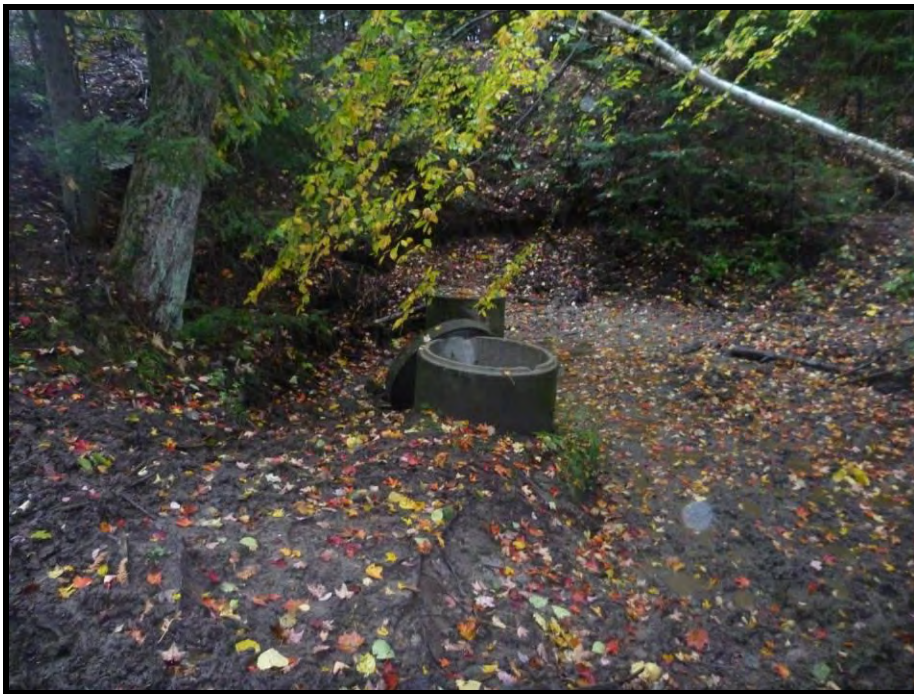
Plate 12: View of Two Cement Wells on Lot 14, Facing West
