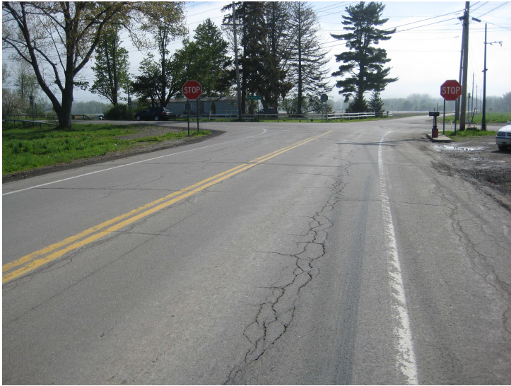
7a. Route 62N, Clear Creek – South Access
