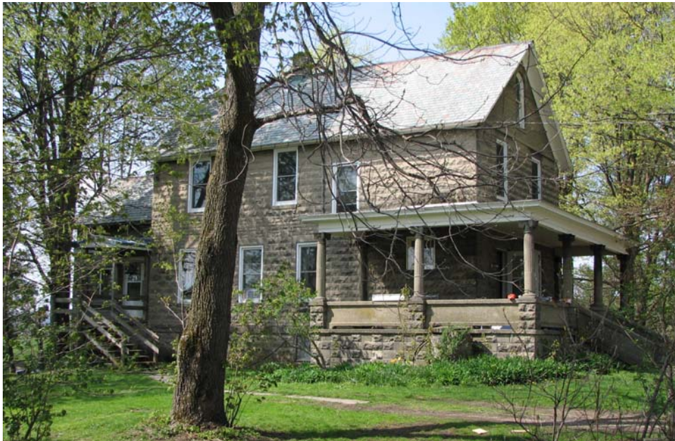
Photograph 4.15. The best example of the Rusticated Concrete-Block house in the study area, this structure, ca. 1920, is located at 8143 Oaks Road, Town of Dayton, Cattaraugus County ( Panamerican 2008 ).
