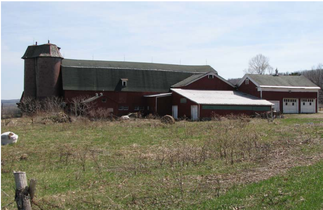
Photograph 4.26. An excellent barn complex at 8911-8903 Farrington Hollow Road in Blacks Corners. It is the original farmstead in the hamlet. The complex consists of several barns, the earliest of which is a Greek Revival, ca. 1850. The long gambrel roof barn, ca. 1900, has three tile silos attached under one roof. It was completed in 1936 and, according to the owner, was the first one of its kind in Chautauqua County ( Panamerican 2008 ).
