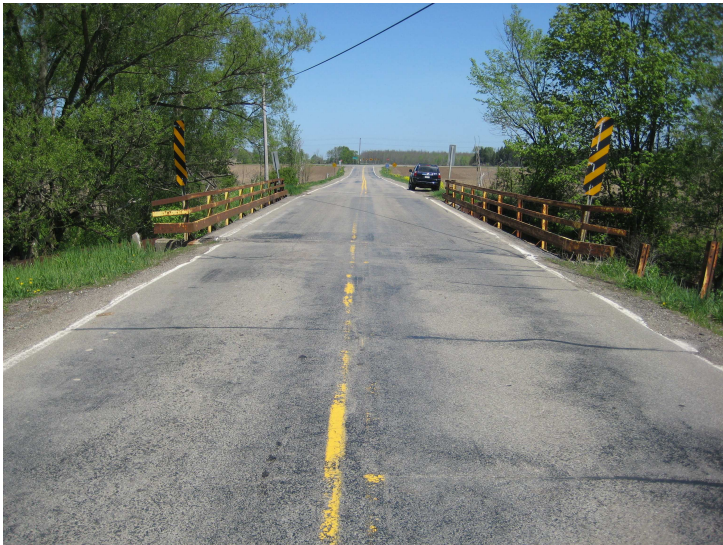
14c. Balcom Cross Rd Bridge Looking North
