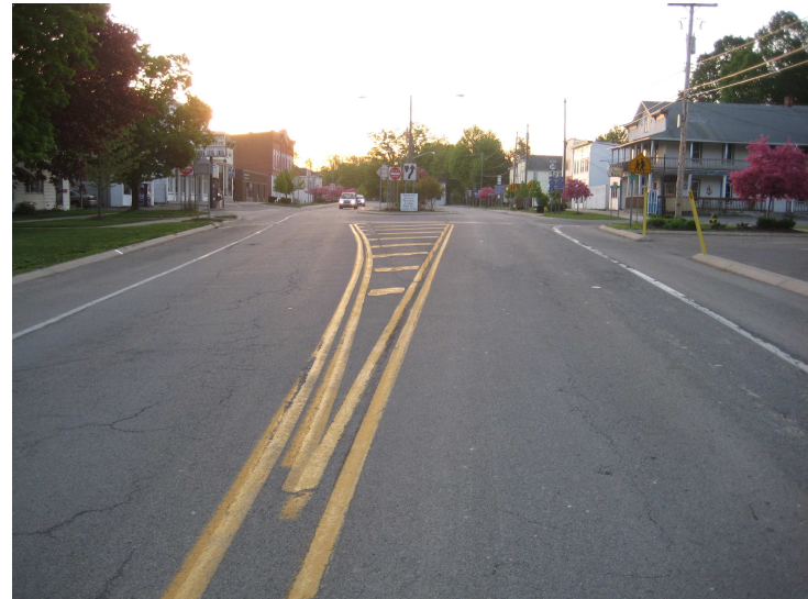
9d. Route 39E Forestville Center – NW Access
