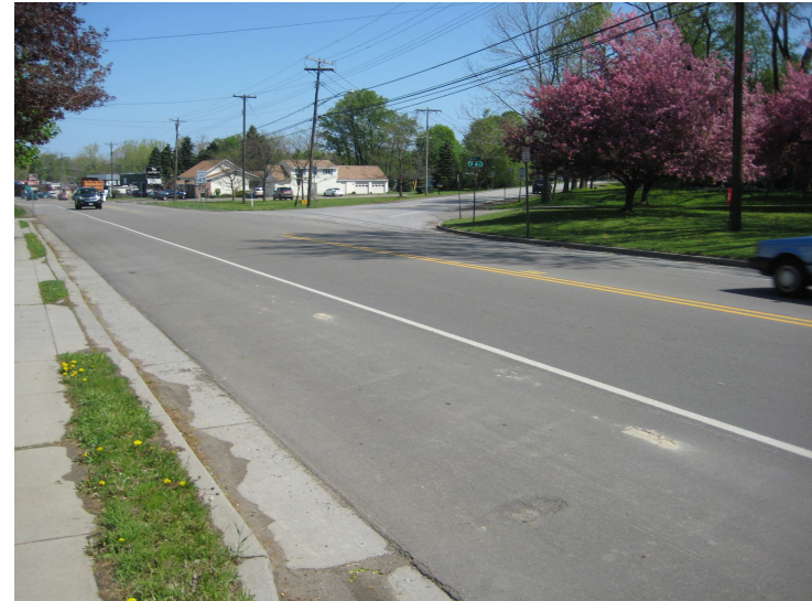
8b. Route 60 at CR 72, Looking East – SW Access
