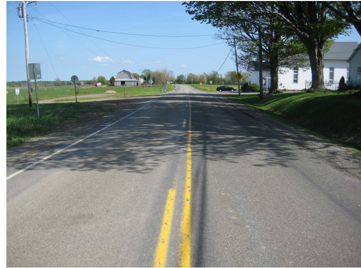
16b. Ball Hill Rd at Bartlett Hill Rd Looking South
