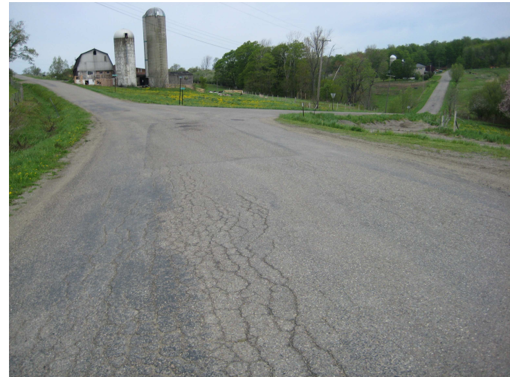
16d. North Hill Rd at Pope Hill Rd Looking North
