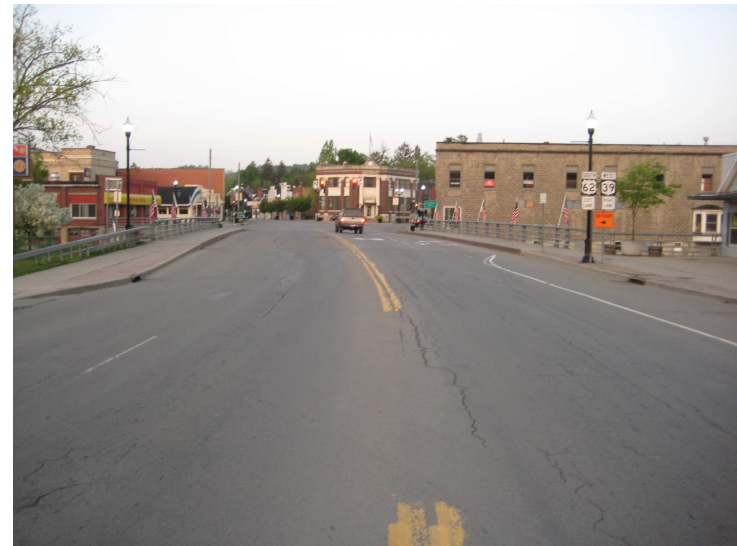
4d. Gowanda Bridge over Cattaraugus Creek
