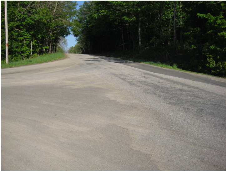
11a. Empire Rd at Hurlbert Rd Looking East
