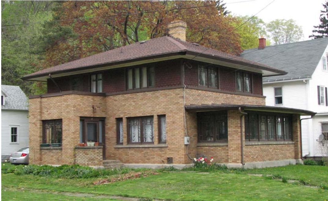
Photograph 4.19. The property at 27 Parkway Avenue, ca. 1915, in the Village of Silver Creek, Town of Hanover, is a rare, excellent example of a Prairie-style residence in the study area. ( Panamerican 2008 ).
