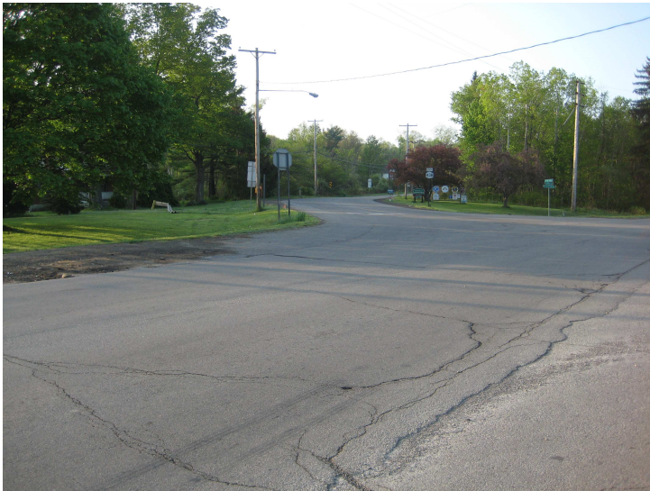
3c. Taylor Hollow Rd at Route 438S Looking South
