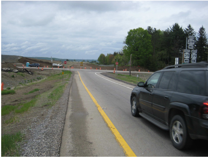
1a. End Route 219S at Route 39, Springville, NY
