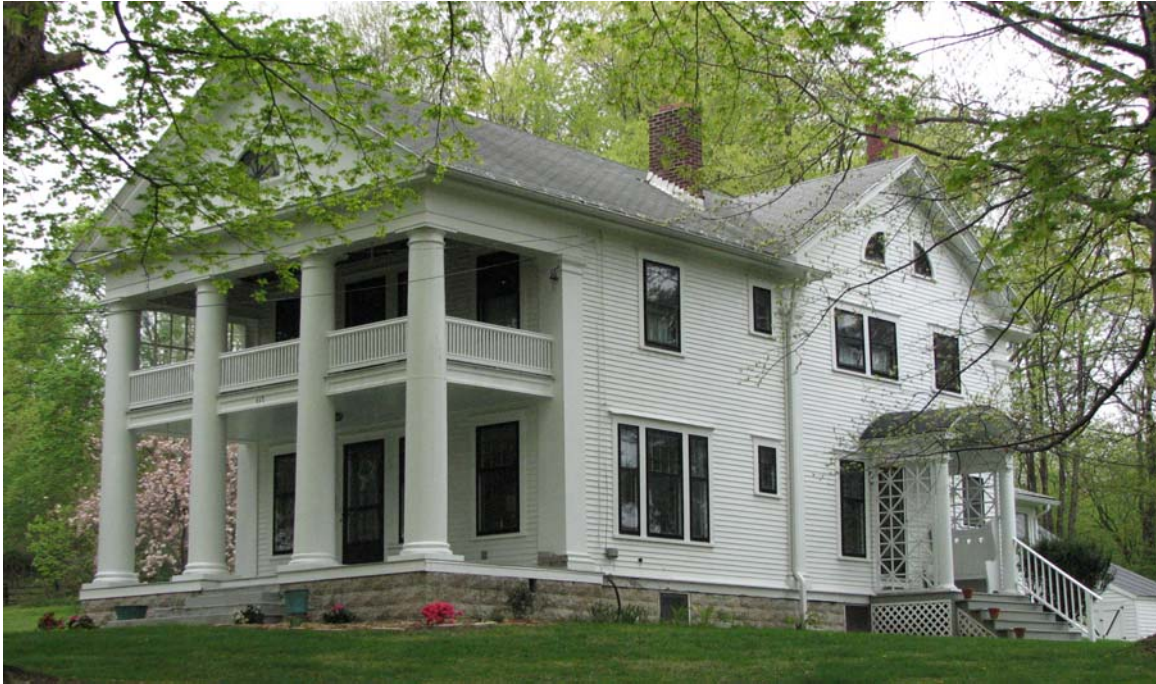
Photograph 4.18. An excellent example of a Neo-Classical residential dwelling, ca. 1920, is the building at 117 Old Main Street in the Village of Silver Creek. It features full height Doric columns, second story balustrade, side pilasters, and full pediment with fan light ( Panamerican 2008 ).
