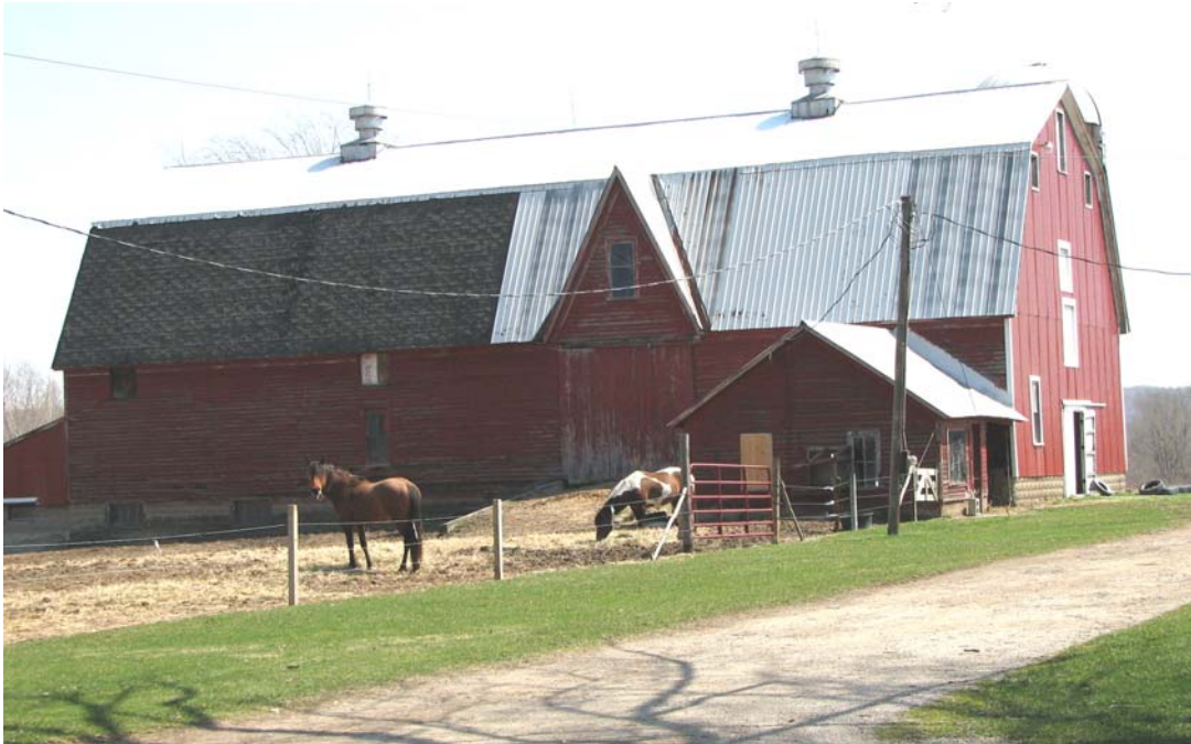
Photograph 4.27. A good example of a gambrel roof bank barn with gabled dormer is located at 8562 NY 83, ca. 1900, in Town of Villenova ( Panamerican 2008 ).
