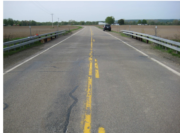
12d. Buttermilk Rd – Small Bridge Looking South
