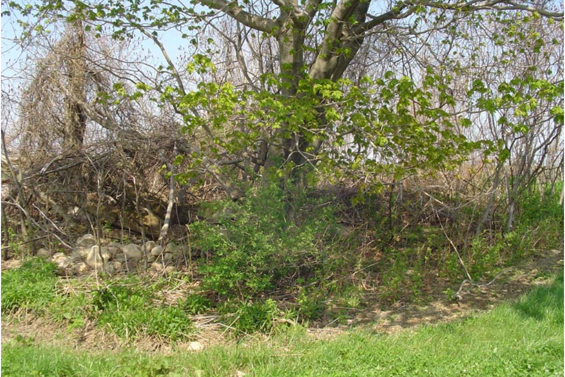
Photograph 17. Close-up of MDS 14 foundation for Linear 14, facing northeast.
