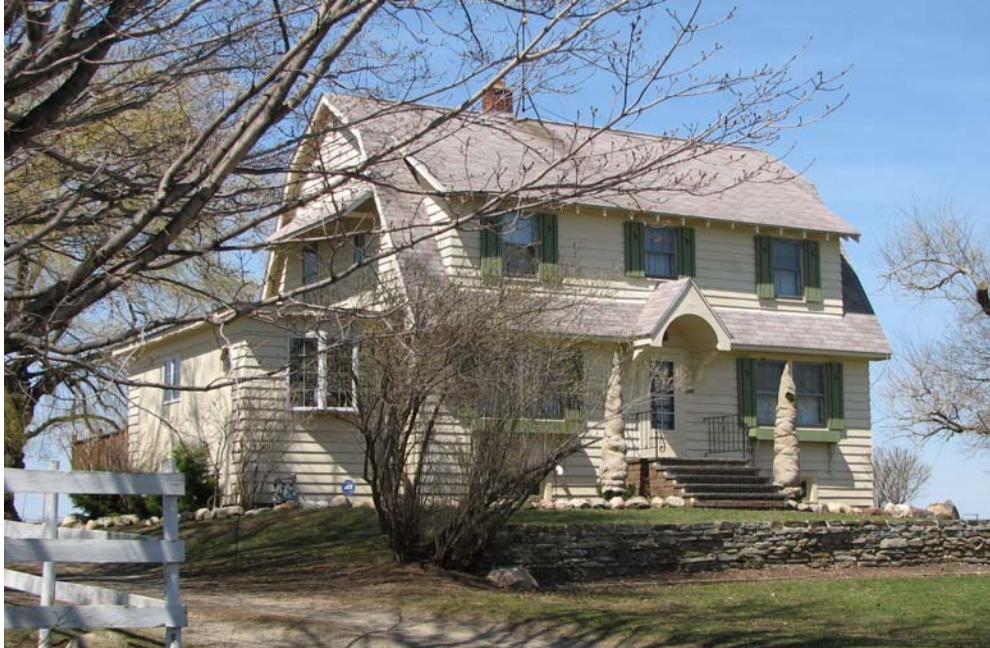
Photograph 4.16. A good example of a Dutch Colonial farmhouse, 1939, is the dwelling at 10292 West Perrysburg Road, Hamlet of West Perrysburg, Town of Perrysburg ( Panamerican 2008 ).
