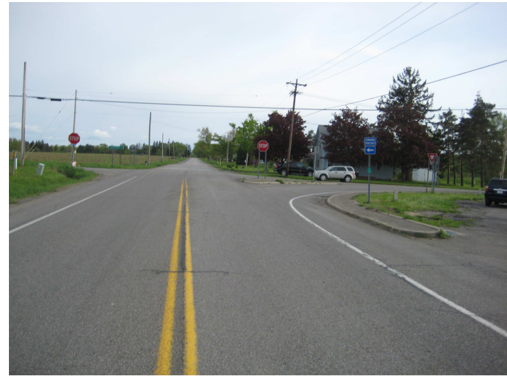
5d. Route 39W at Stafford Rd Looking South
