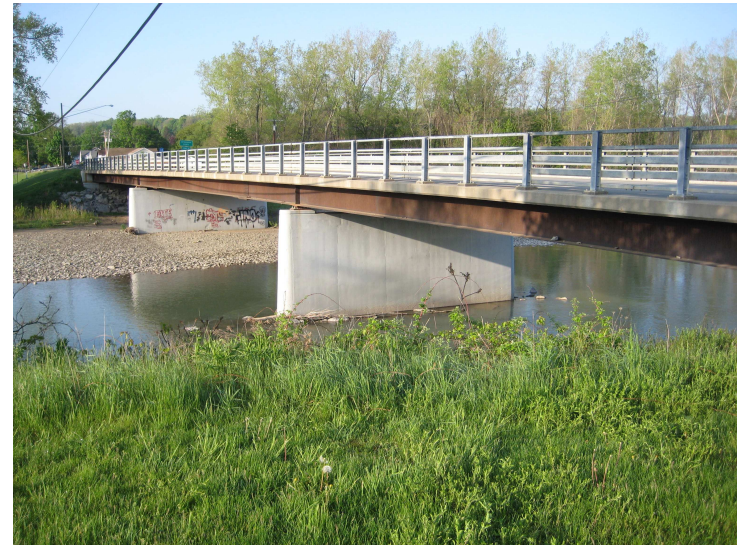
3d. Aldrich St Bridge Looking SW
