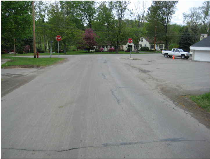
2a. Collins Rd at Route 62 Looking West
