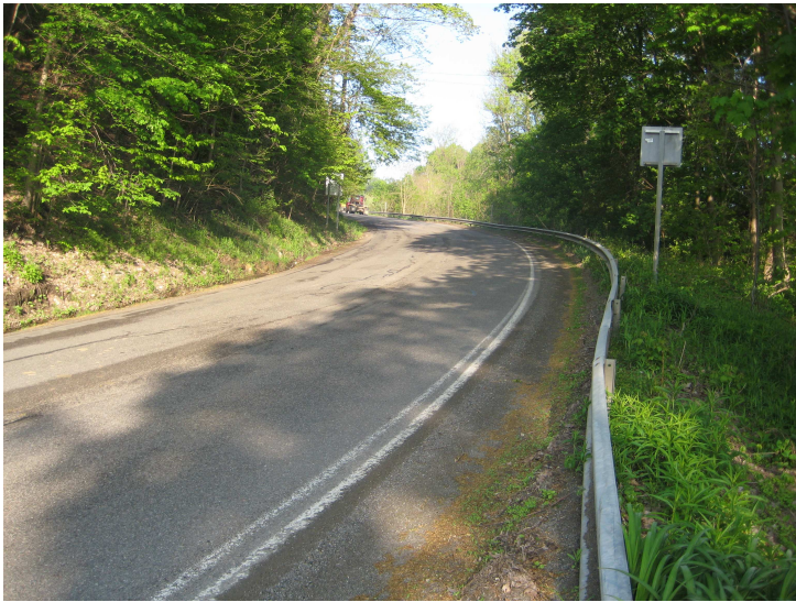
5c. Route 39W – Steep Grades, Perrysburg, NY
