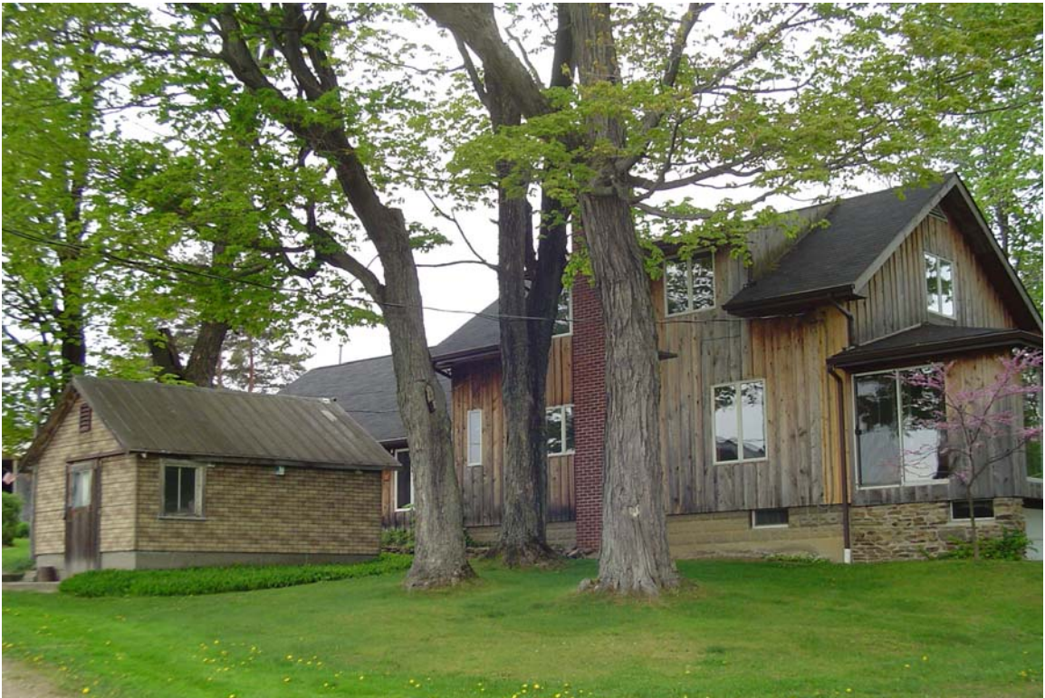
Photograph 18. House located outside the APE of Linear 16, facing southwest.
