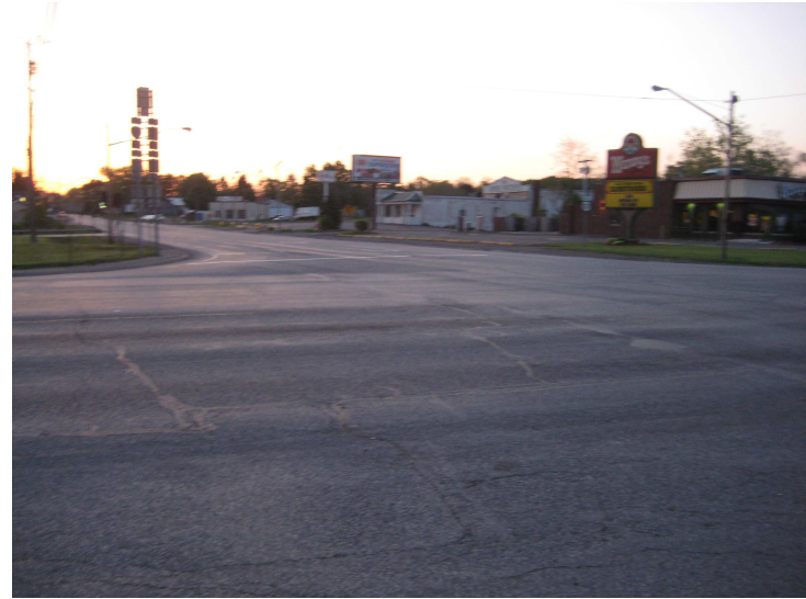
9b. US Route 20E at Route 60 – NW Access
