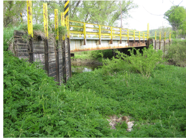
18b. Cemetery Rd Bridge Looking NW
