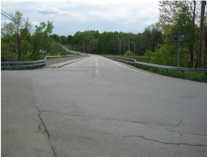
3a. Versailles Plank Rd Bridge over Cattaraugus Creek
