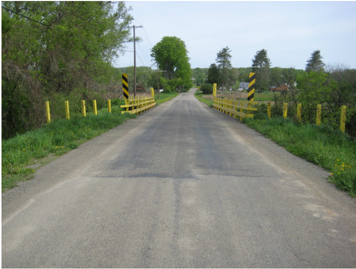
18a. Cemetery Rd Bridge Looking North
