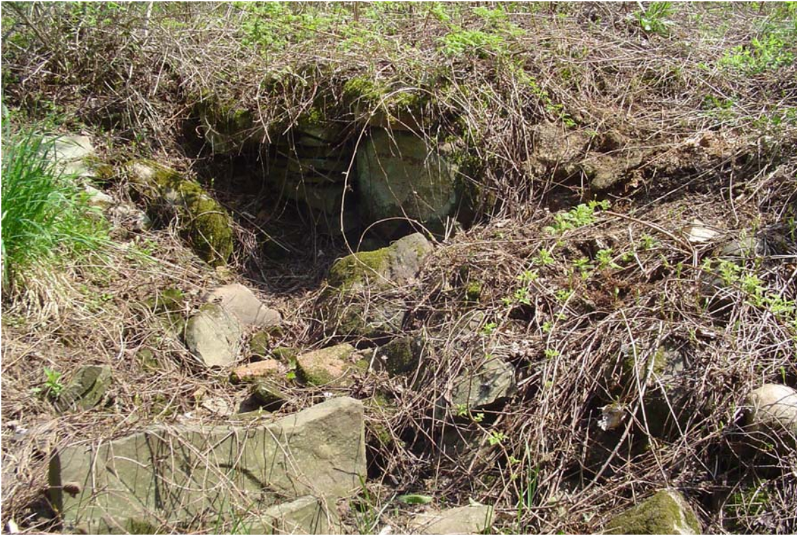
Close-up of foundation at Site PCI/Ball Hill-2, facing northwest.
