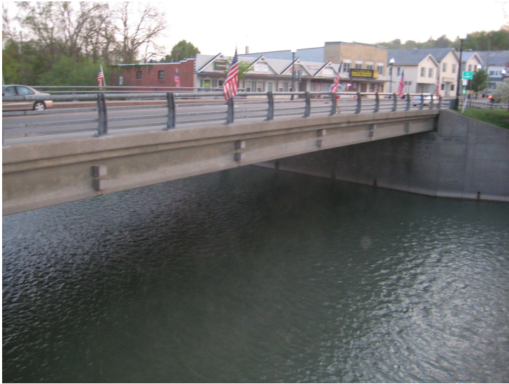
5a. Gowanda Bridge Looking SW
