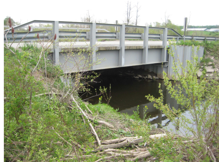
18d. Wentworth Rd Bridge Looking SE
