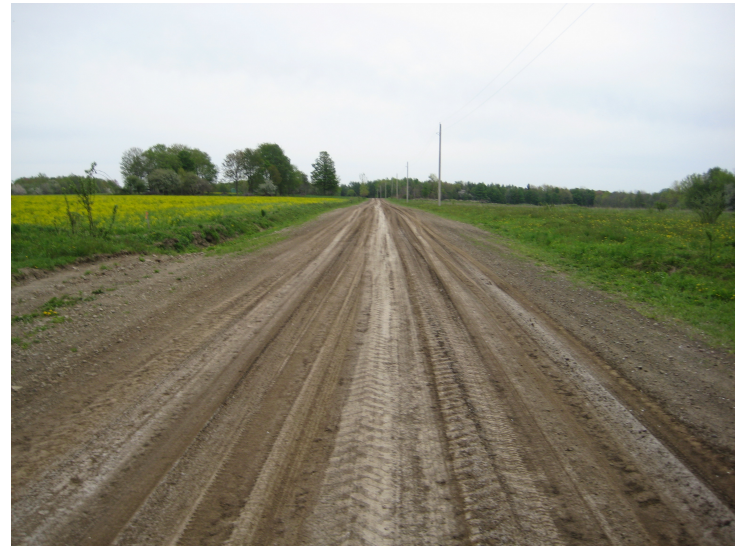
17d. Villenova Rd – Gravel Road Looking East
