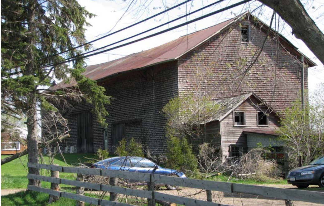
Photograph 4.25. Side gable long barn, ca. 1890, at 7814 NY 83 in the Town of Cherry Creek. The barn maintains its historic wood shingle exterior and clapboard milk house ( Panamerican 2008 ).
