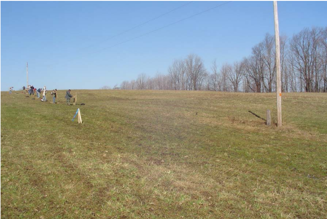
Photograph 4. Overhead power lines and Turbine 2, facing northwest.
