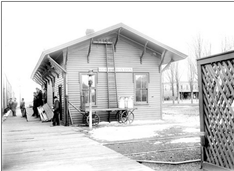
Figure 10.11. South Dayton Depot in 1909 ( Western New York Railroad Archive nd ).
