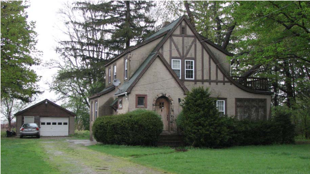
Photograph 4.22. The structure at 11991 Hanover Street, ca. 1930, in Hanover Center, Town of Hanover, is a good example of a Tudor Revival residence. It retains most of its integrity with the exception of new windows ( Panamerican 2008 ).
