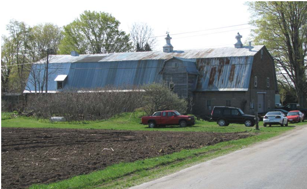
Photograph 4.28. The only gambrel roof bank barn executed in rusticated concrete-block, ca. 1915, in the study area is one that is part of the Dye Homestead at 558 South Dayton-Hamlet Road, Hamlet of Balcom Corners, Town of Villenova ( Panamerican 2008 ).
