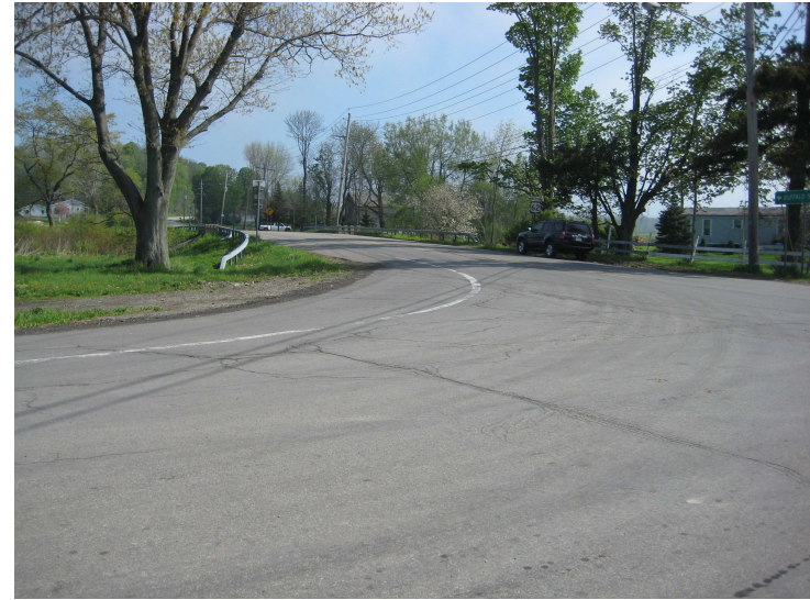
7b. Route 62N, Clear Creek, Looking North
