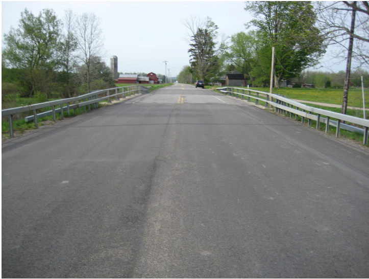
12a. Buttermilk Rd – Big Bridge Looking South
