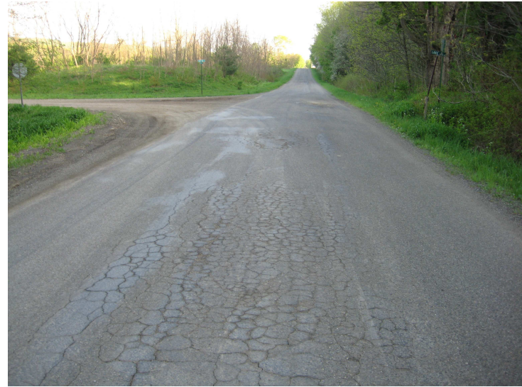
11b. Dye Rd at East Lake Rd Looking South
