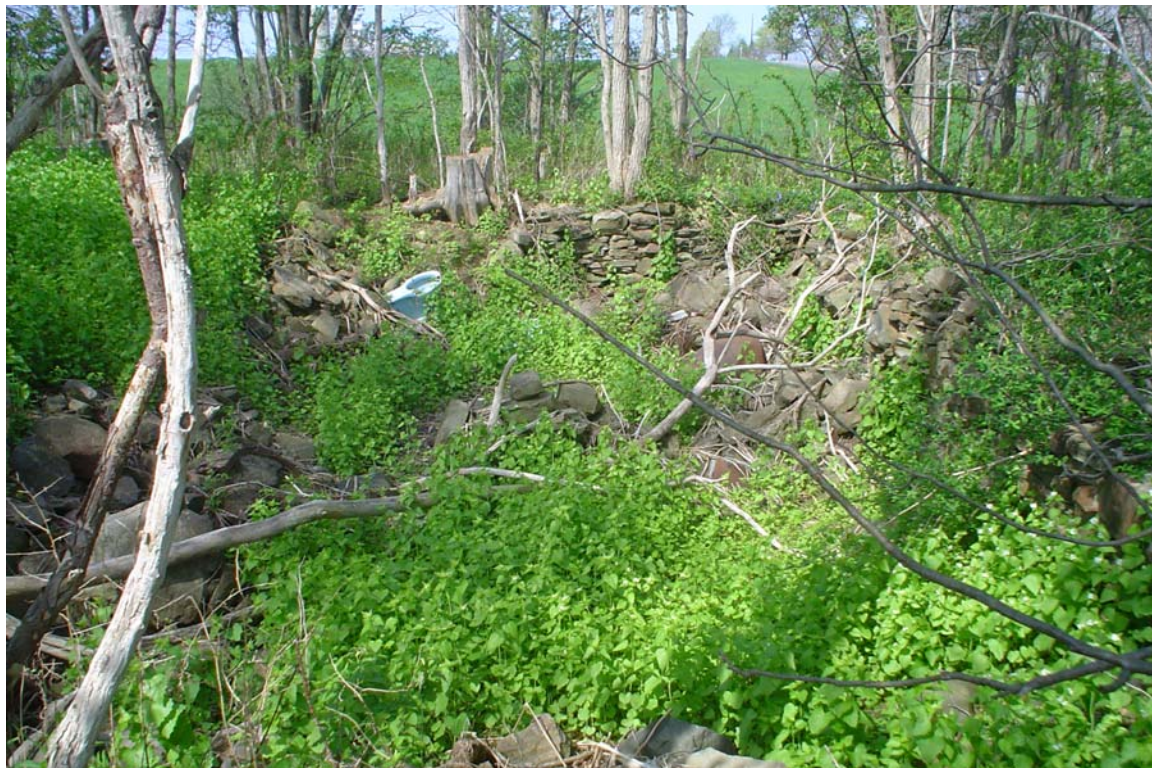
Foundation at Site PCI/Ball Hill-1, facing west.
