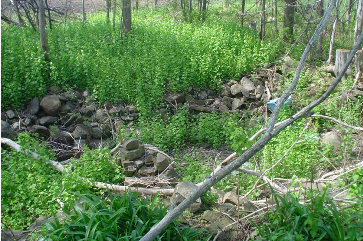
Close-up of foundation at Site PCI/Ball Hill-1, facing southwest. Note: central pile of stones represents footer (approximately 2ft by 2ft [6.5 m x 6.5 m]) for a fireplace or central floor support.
