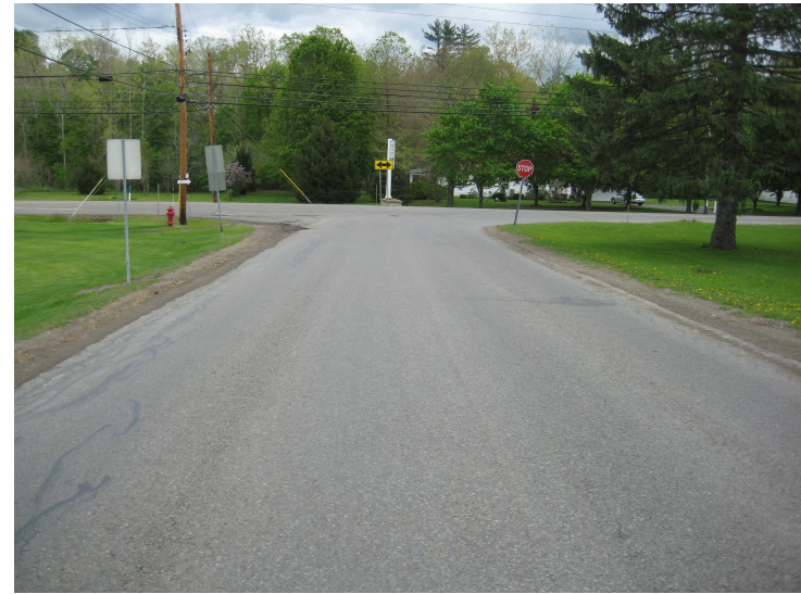
2d. Richardson Rd at Route 62 Looking East
