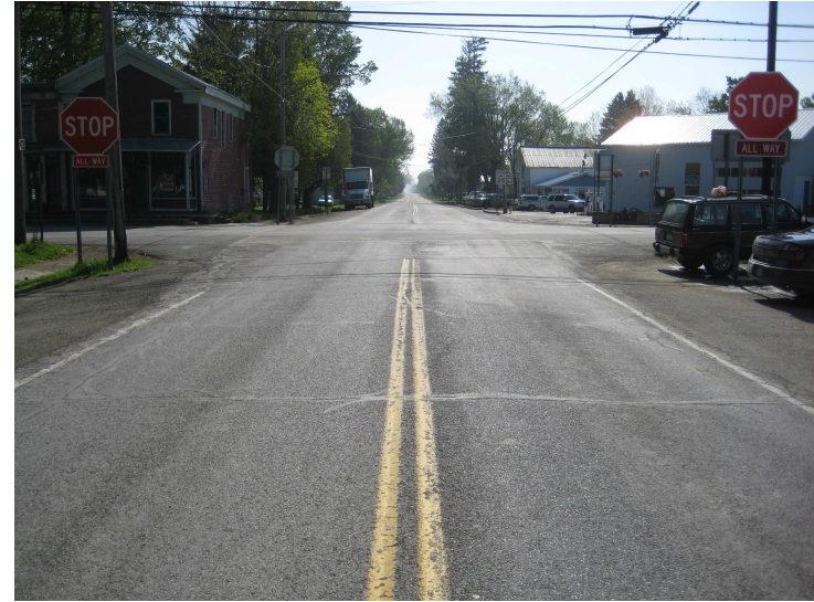
6d. Route 62N, Ellington Center - South Access
