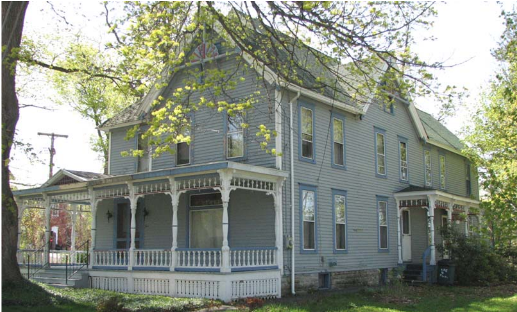
Photograph 4.13. A largely intact example of a Queen Anne-style residence, ca. 1890. It is one of the most intact Queen Anne structures in the study area. Found at 4 Pearl Street in the Village of Forestville, the building is in the negative viewshed ( Panamerican 2008 ).
