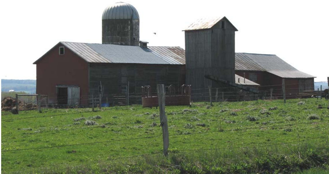
Photograph 4.29. A side gable long barn with modern concrete silo and frame square silo, is located at 8052 NY 83 in the Town of Villenova ( Panamerican 2008 ).
