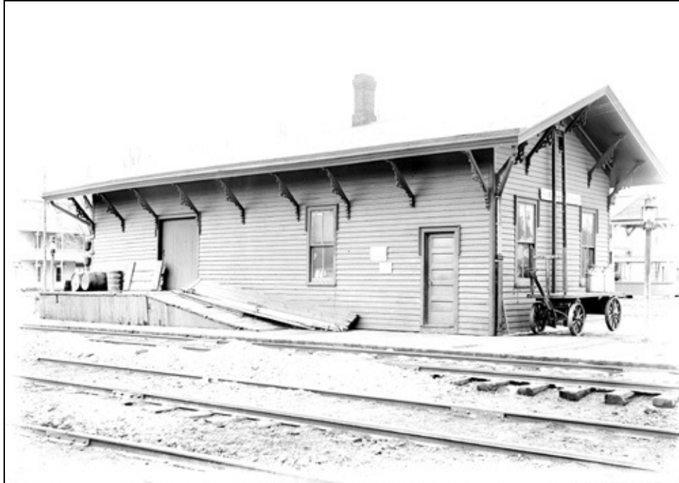
Figure 10.4. South Dayton Depot in 1909 ( Western New York Railroad Archive nd ).
