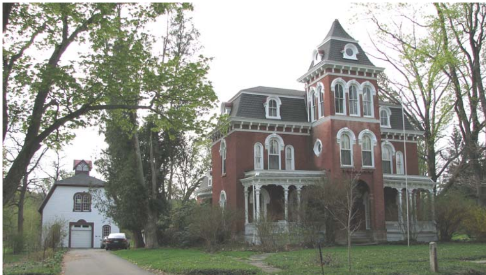
Photograph 4.11. An excellent example of a high style Second Empire-style residence, ca. 1880, located at the intersection of Pearl and Center streets in the Village of Forestville. Found in the negative viewshed, the building features: symmetrical massing, full width porch, center tower, rounded arched windows with hoods, bracketing under the mansard roof and mansard roof tower with oculus windows ( Panamerican 2008 ).
