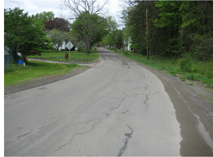
1d. Collins Rd By-Pass Looking West
