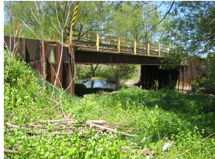
14d. Balcom Cross Rd Bridge Looking NW
