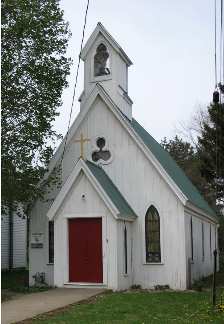
Photograph 4.7. A highly intact Gothic Revival Church, ca. 1850 located on Park Street in the Village of Forestville. This building is situated in the negative viewshed (Panamerican 2008).
