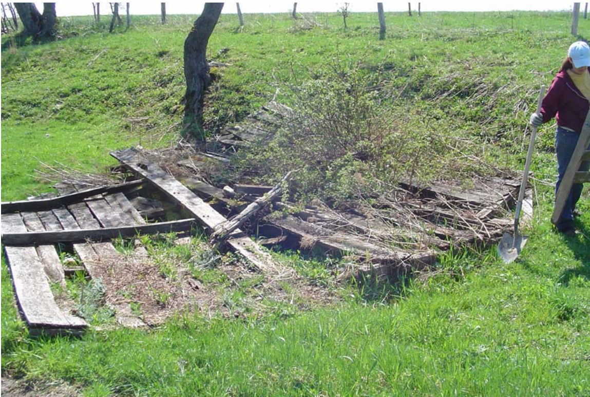
Photograph 12. Wood pile at Turbine 46, facing southeast.
