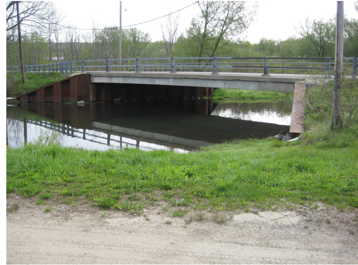
12b. Buttermilk Rd – Big Bridge Looking SW
