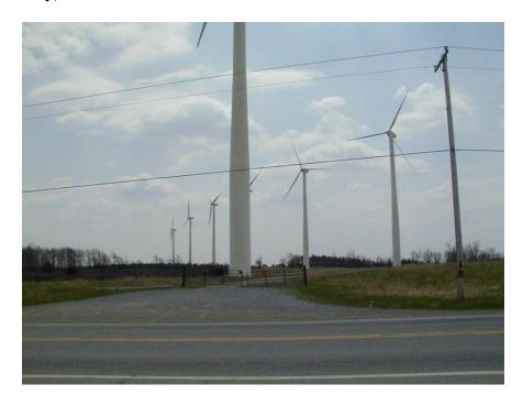
The Wethersfield Wind Farm is a 10 turbine, 6.6 MW wind energy farm located in the Town of Wethersfield, in Wyoming County, New York. The 310 acre Wethersfield site is located along one of the highest ridges in Wyoming County. The wind energy project came online in October 2000. The site consists of ten (10) 213-Foot High turbine towers & 154 foot rotor diameter. Total turbine height is 290 feet.
