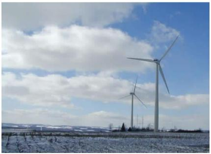
The Madison Wind Farm is located in the Town of Madison, Madison County, New York. This project was New York's first commercial wind farm and has been on line since September 2000. The site consists of seven (7) 220-foot high turbine towers & 216-foot rotor diameter. Total turbine height is 339.25 feet.
