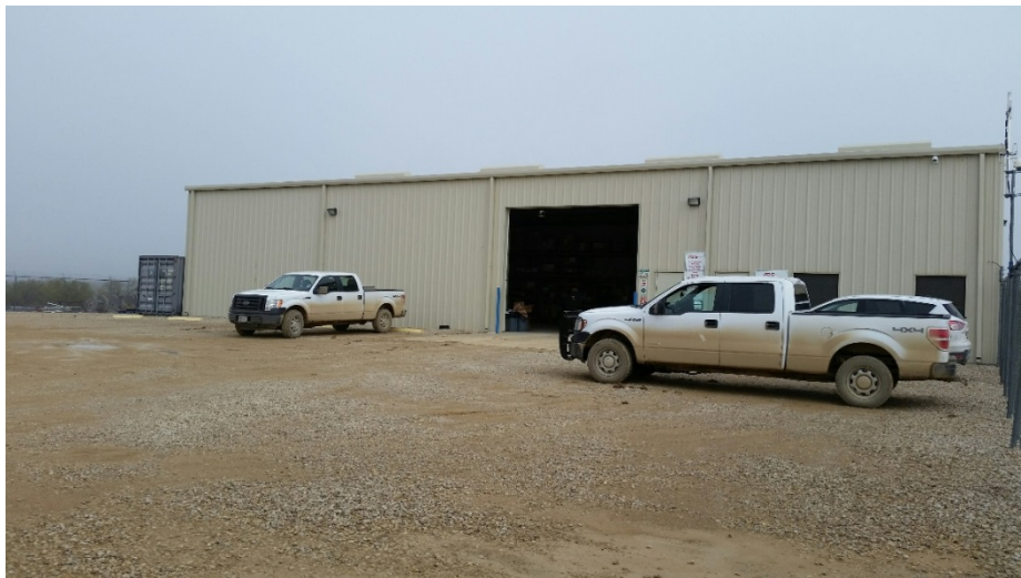
Typical O&M Building (back)
