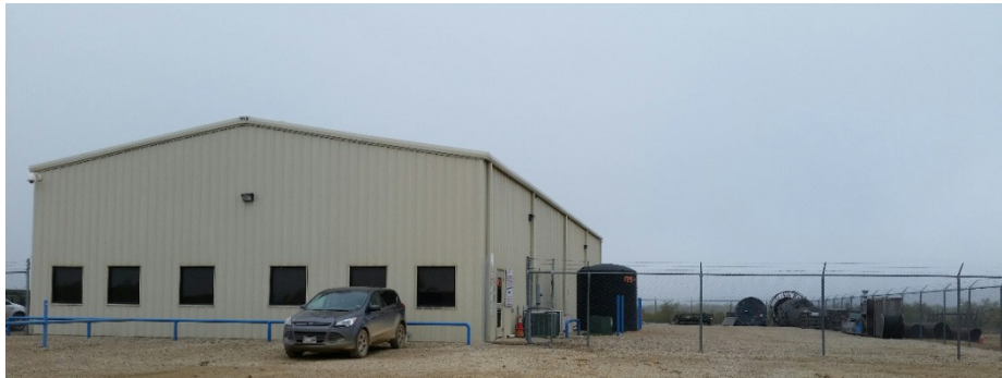
Typical O&M Building (front)
