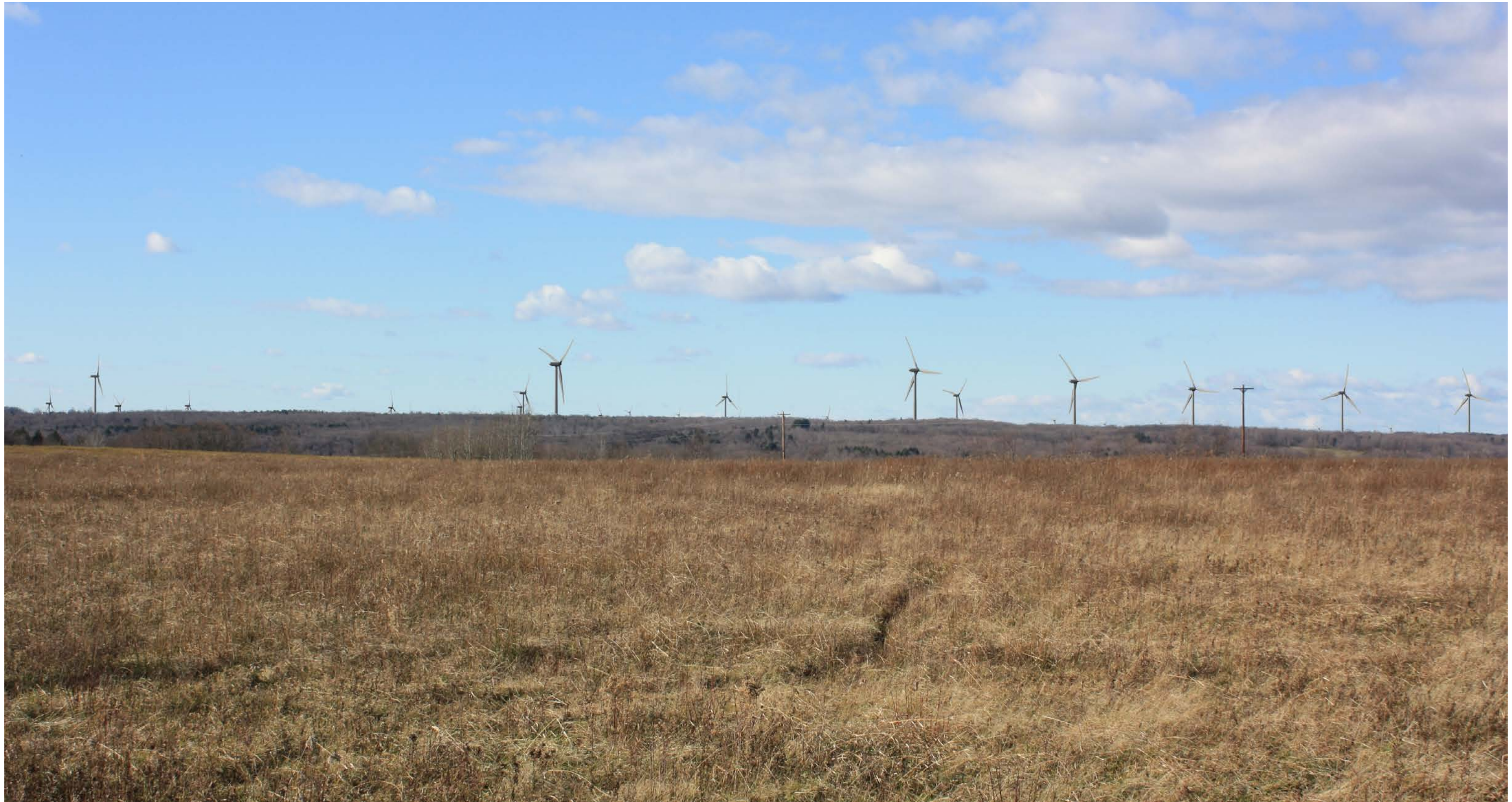
Proposed Condition - Ball Hill Wind Project, Arkwright Summit Wind Farm and Cassadaga Wind Project
