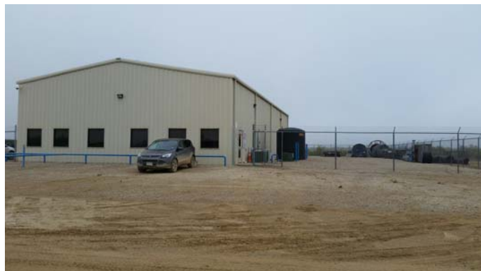
Typical O&M Building and Side Yard
