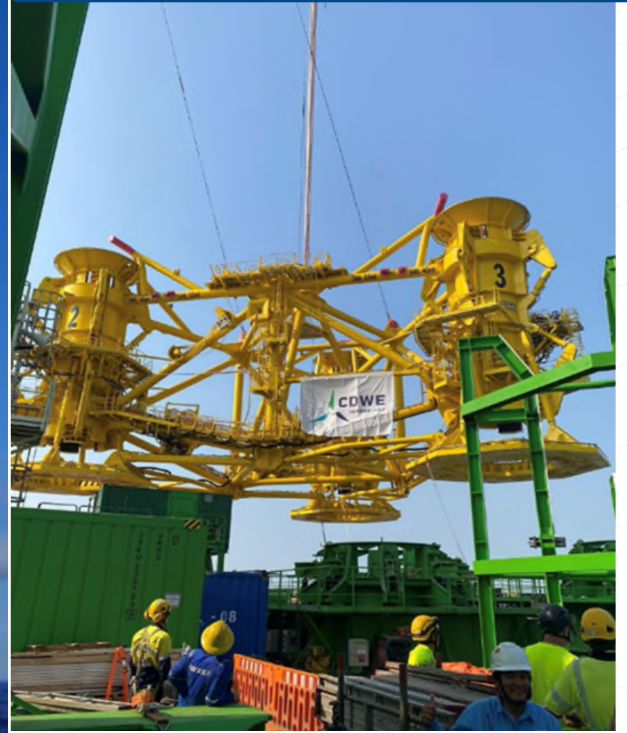
Load out of piling frame in Vietnam, February 1st, 2024
